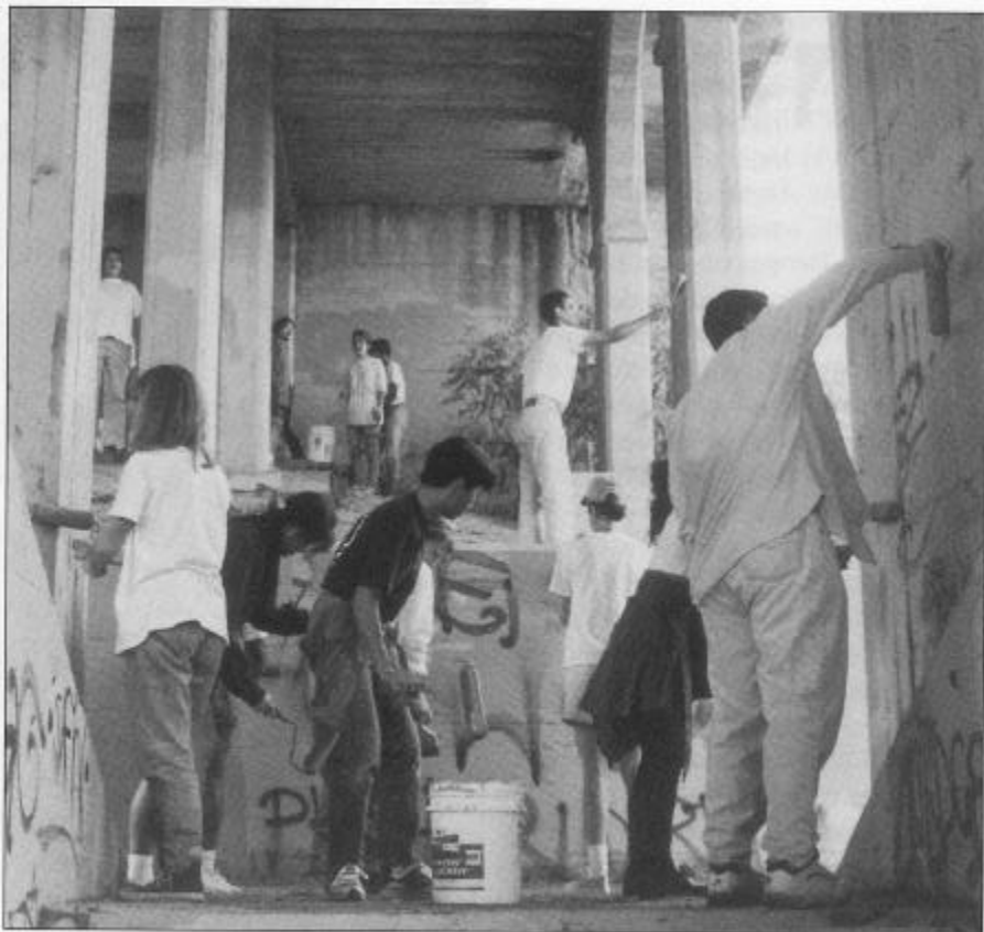
Students at La Sierra University (Riverside, California) remove graffiti from a local bridge during Community Service Day, 1994.
