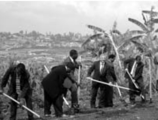
Groundbreaking for a new campus at Adventist University of Central Africa (AUCA) in Rwanda.
