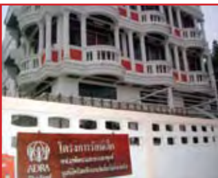
The KGS house in Chiang Rai has offices, kitchen, worship room, and accommodation for 50 girls. ADRA headquarters and a board room are on the top floor, and out back are fields for growing rice and vegetables.
